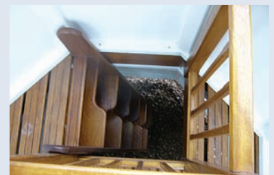
A space saving 'paddle stair' inside the lighthouse
